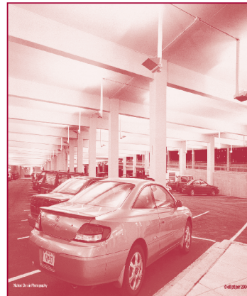
Uplighting on structure ceiling
